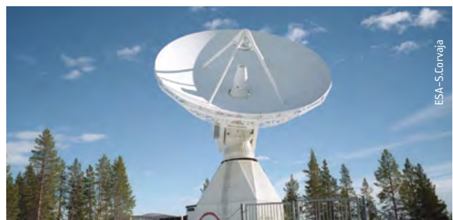
The Kiruna S- and X-band station is located at Salmijärvi, 38 km east of Kiruna, in northern Sweden
